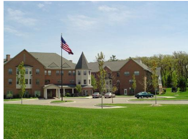
2001 Mendelson Home -- 60 assisted living apartments for the frail elderly.
